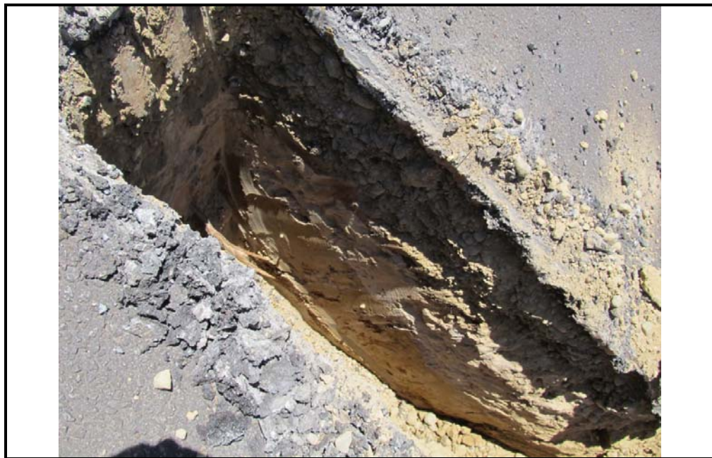
Photo 12: Photograph of roadbase fill profile on access road – eastern Lot 418.
